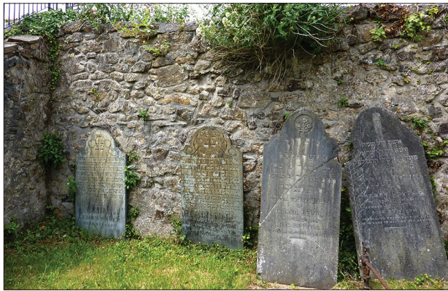
Wall restoration - The northwest back inner wall of the Penzance cemetery which will soon be restored to its former splendour.
